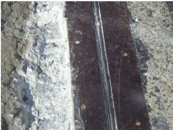
Joist Before Blast
