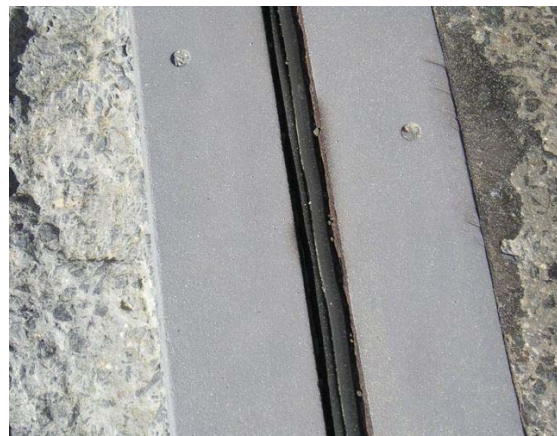
Joist After Blast
