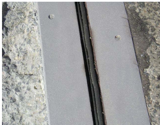
Joist After Blast
