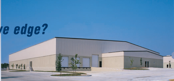
AERCON panels were selected for cladding on this 25,000 sq. ft. warehouse.
