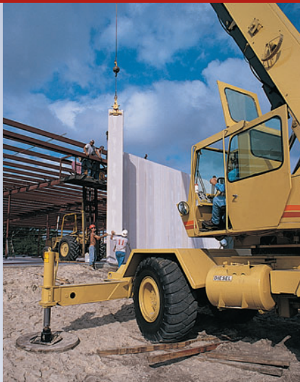
Industrial warehouse cladding installation.
