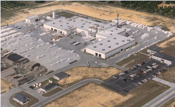
AERCON's manufacturing facility is located in Haines City, Florida.
