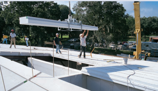
Roof Panel installation completed in one day.
