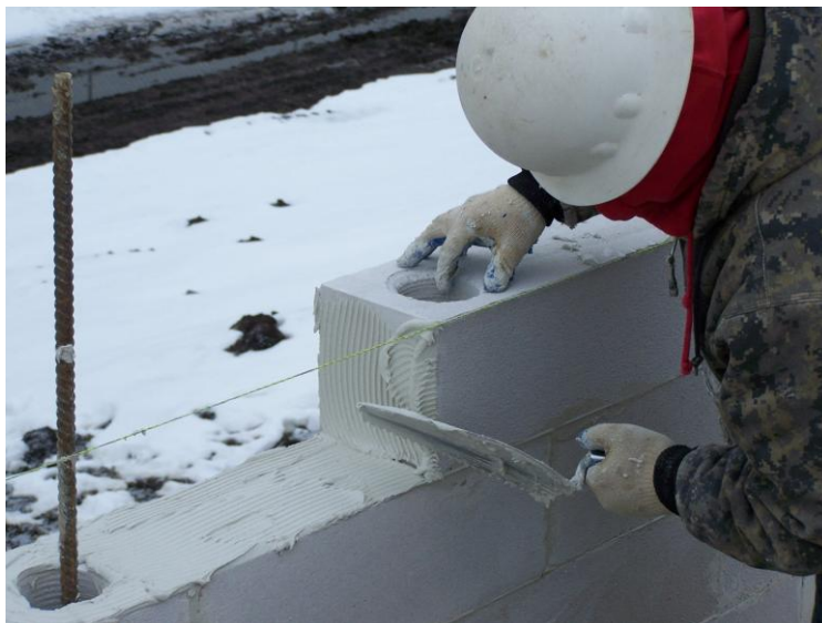
Figure 8. Bricklayers use a notched trowel and thin-bed mortar to bond AAC units together.
