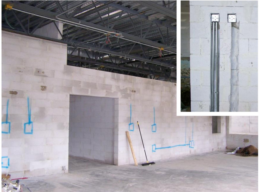
Figure 10a. Electricians marked locations for their conduit and boxes on the AAC; bricklayers routed electrical chases into the AAC for recessed conduit and boxes (inset).
