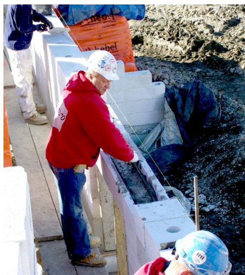
Figure 4. AAC bond beams provide rigidity to transfer lateral and gravity loads.
