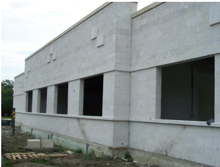
Figure 10b. AAC appliqué were adhered to the walls to form a projected soldier header course, a rowlock sill, and projected medallions, all to resemble clay brick after the coating is applied.
