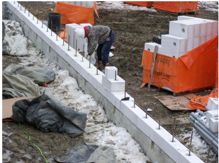
Figure 7. Leveling course was laid in Type S mortar; top of fdtn. is notched for recessed conduit; #5 fdtn. dowels @ 24-in. o.c. line up w/ pre-cored AAC units.
