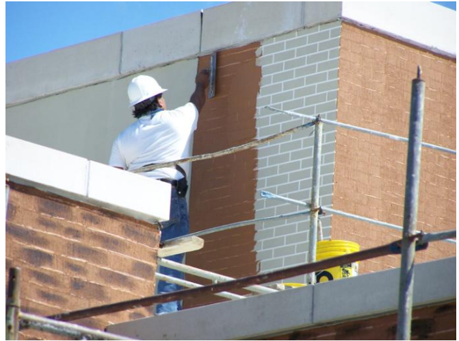
Figure 11a. DEFS is applied in three coats, with the final product matching the brick color on the existing Village Hall building.
