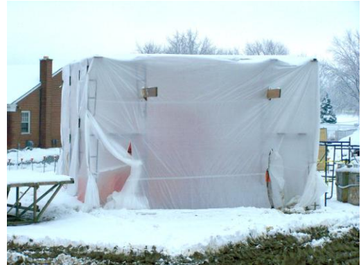
Figure 6b. Heated enclosure for staging material.
